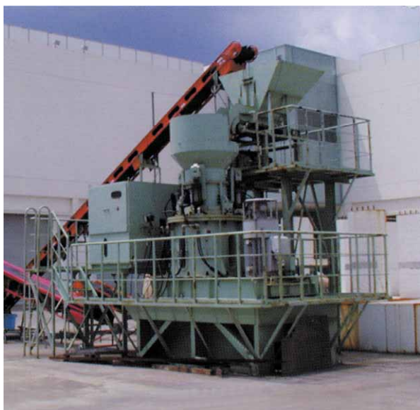
図2 設備全景 Fig. 2 Whole view of equipments
