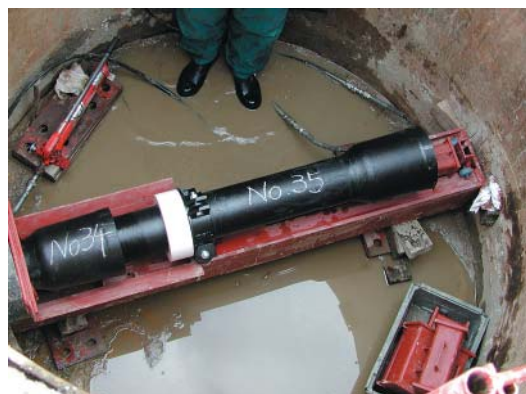
図11 施工状況 Fig. 11 State of construction
