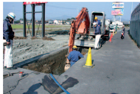
図7 掘上げ状況 Fig. 7 State of digging test pipes
