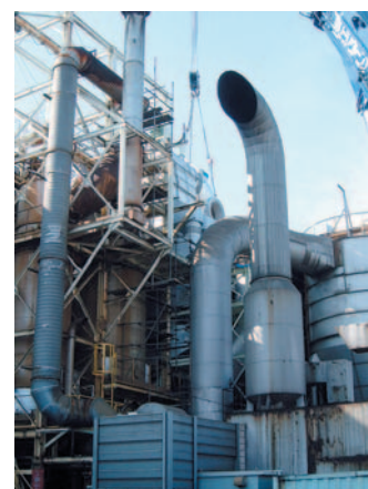
図7 空気予熱器更新工事 Fig. 7 Renewal construction of the recuperator
