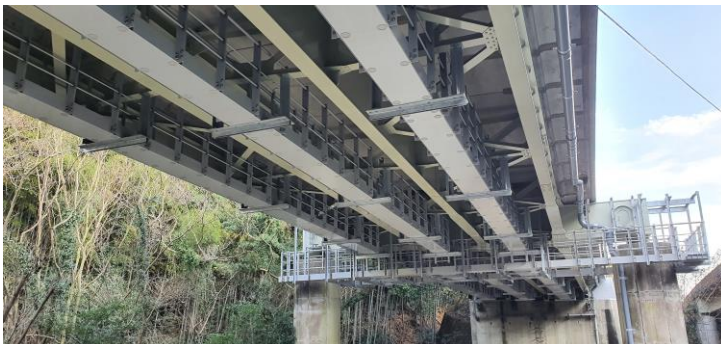
Yamanaka Viaduct, Kanmon Expressway
