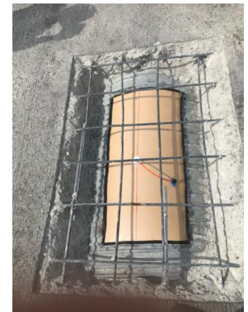
4. Completion of installation
