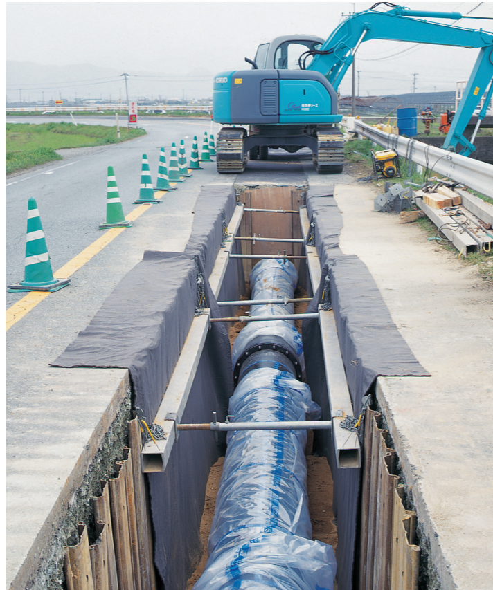
Polyethylene sleeves being used to protect Ductile Iron Pipe.
